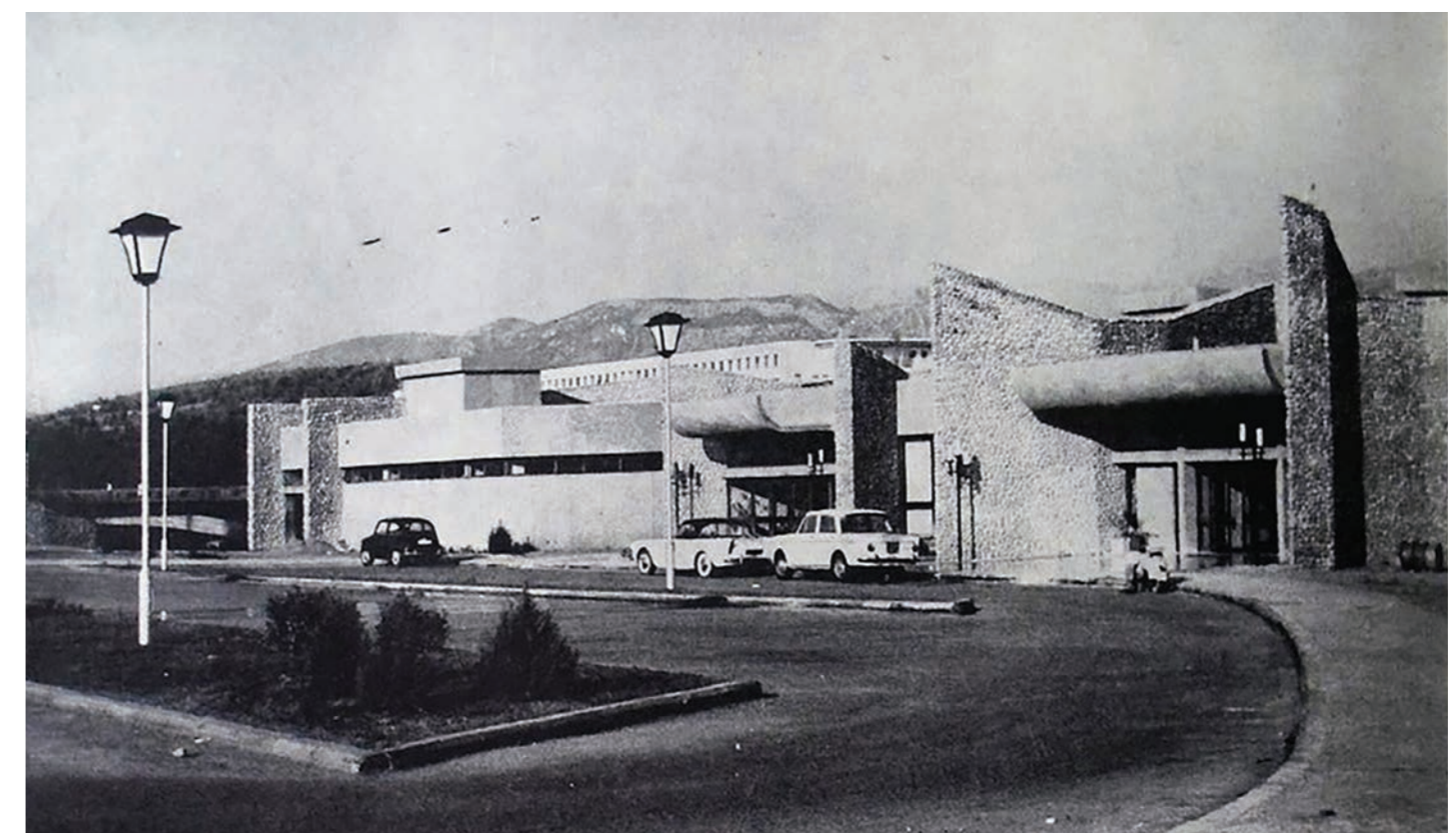
The main entrance of Hotel Podgorica, North West facade, after finishing the construction 1967.
