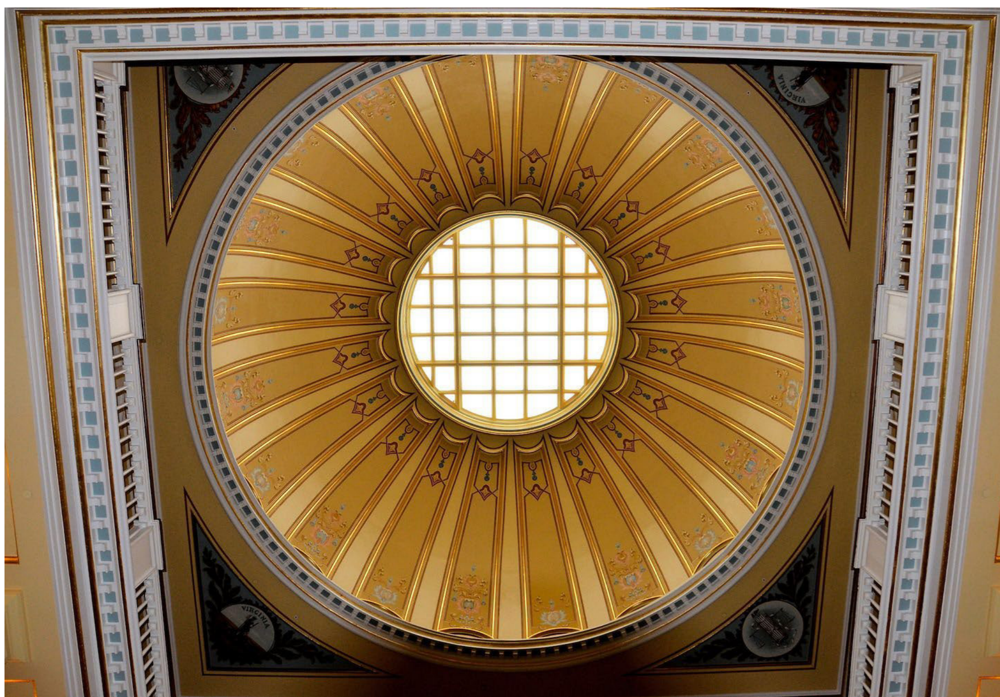
A gold lined internal dome located within the Virginia Statehouse, peering down upon the statue of George Washington
